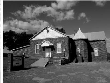
Flat Rock Church of the Brethren Limestone Road Forestville, Virginia
